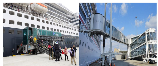
Fig. 2. Cruise ship's passenger boarding bridge.
