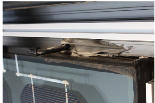
Fig. 1 Wiring hole processing example
