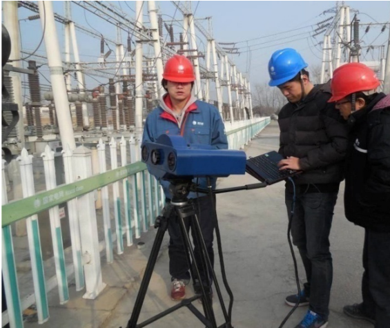
FIG. 12. Experimental scene in the Sunjiashai 110 kV substation which is located in Qinghai Province of China.
