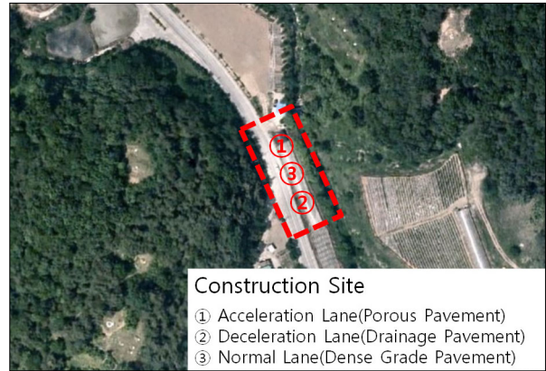
(a) Construction Site
