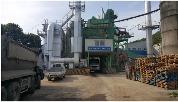
(a) Asphalt Mixing Plant
