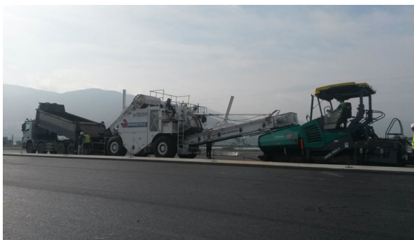
Fig. 1 Asphalt Paving with MTV
