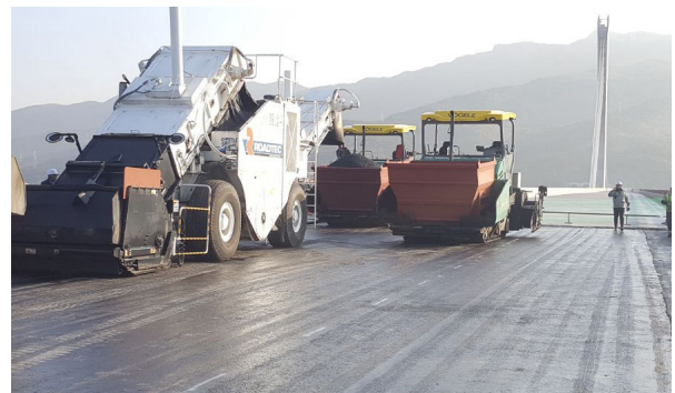
Fig. 2 Simultaneous Material Supply from a MTV to Two Finisher
