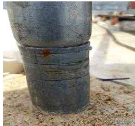
Fig. 6. Work fixing the column.
