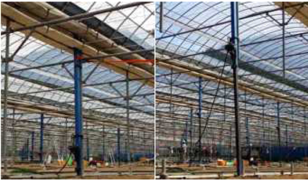
Fig. 7. Before and after construction.
