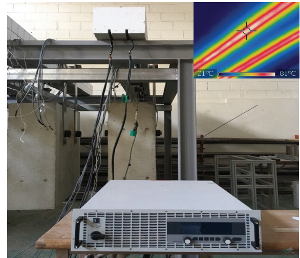
Fig. 5 Activation of NSM Fe-SMA strips
