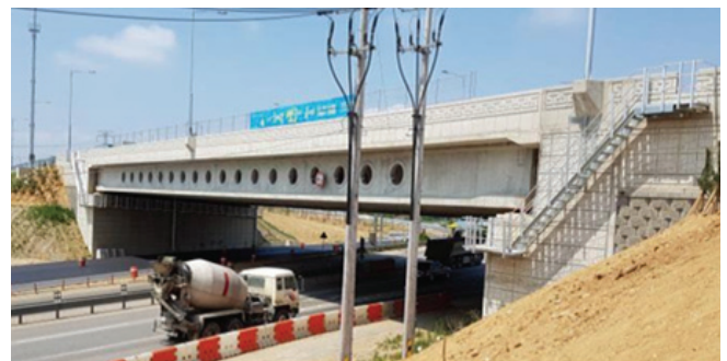
Fig. 3 View of The Bridge
