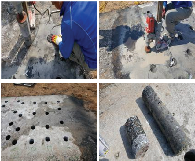
Fig. 6 Mock up coring
