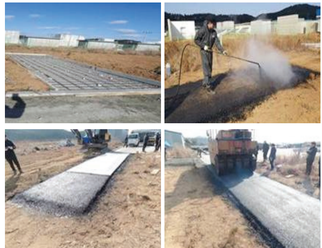
Fig. 5 Mock up construction
