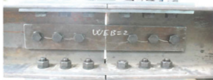
Photo 13 Situation after Existing Joint Test
