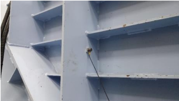
Fig. 7 One-axis accelerometer for vibration measurements
