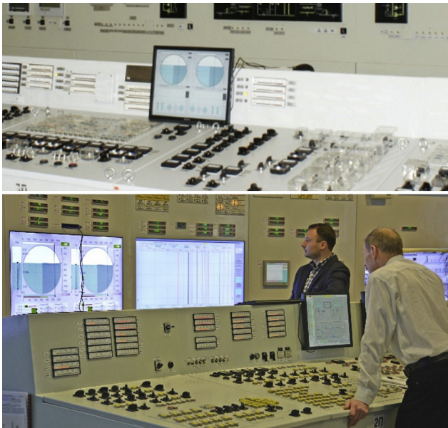
Fig. 8. Testing of the ecological display at LNPP (upper photo) and SNPP (lower photo). LNPP, Leningrad NPP; SNPP, Smolensk NPP.
