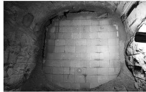
Fig. 16. The installation of the full-scale backfill at the Aspö HRL.
