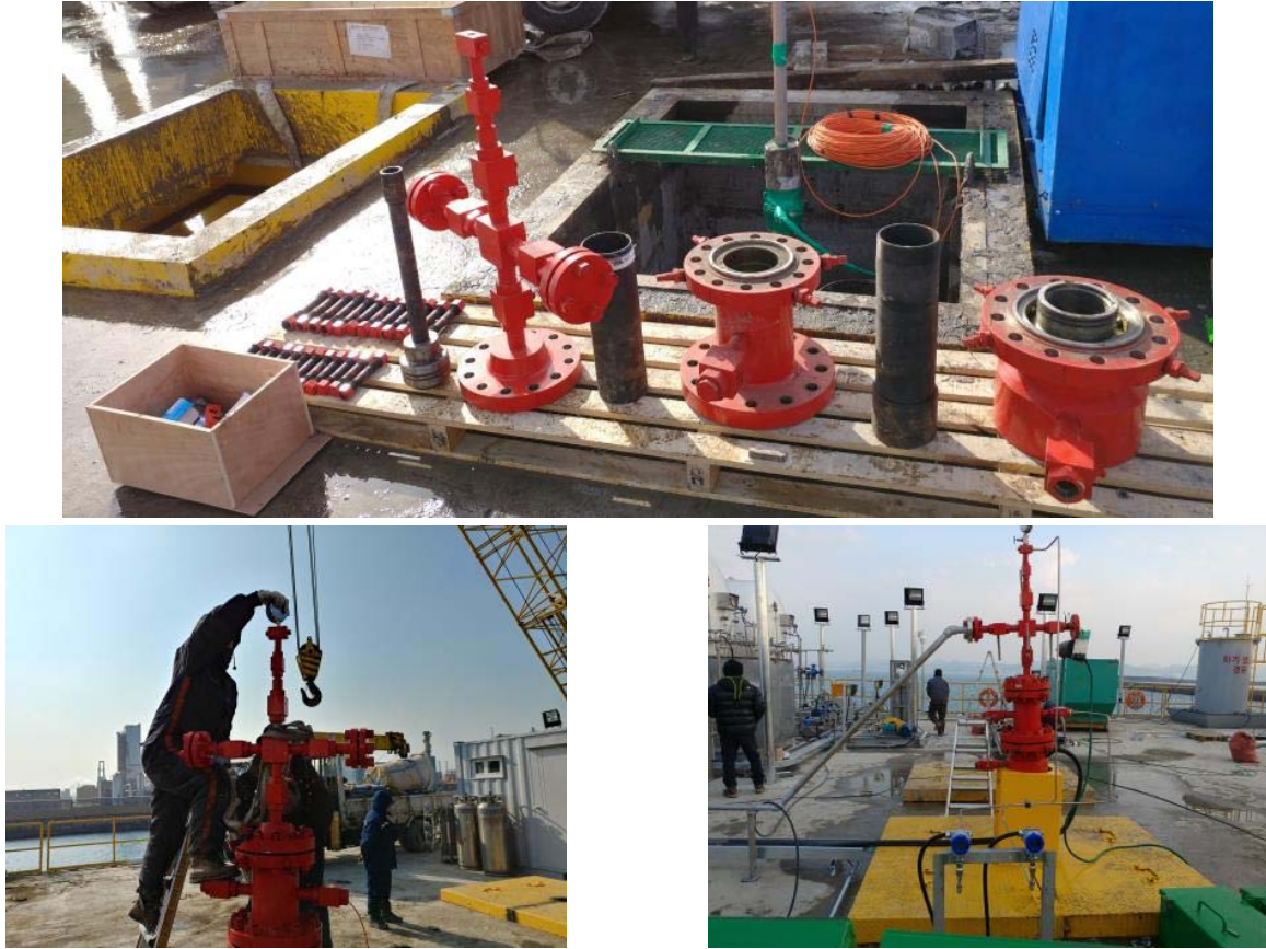
Fig. 11. Installation process of the christmas tree and wellhead.
