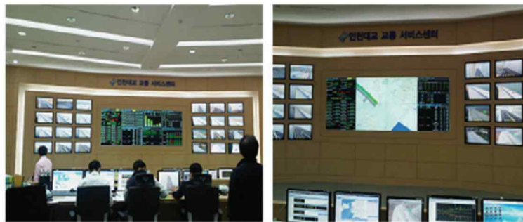
Fig. 11. Road Weather Information System Management Center in Incheon Bridge
