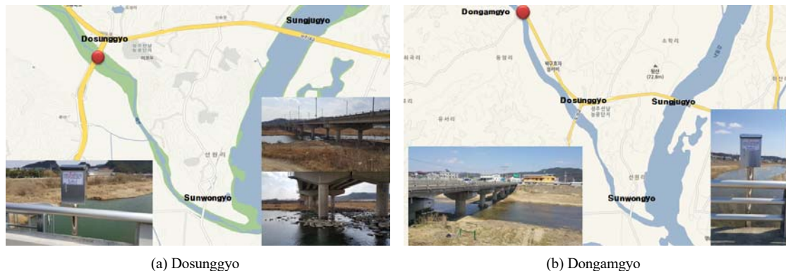
Fig. 3. Water level gauge installation.
