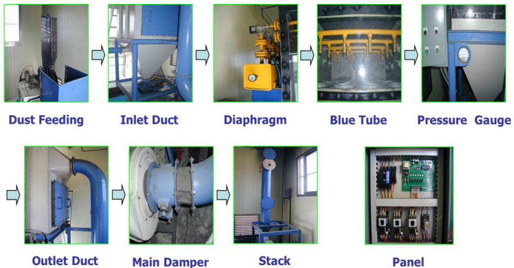
Fig. 2. Removal procedure of the coke dust.
