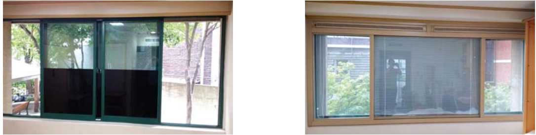
Fig. 3 Existing window (left), Retrofit window (right)
