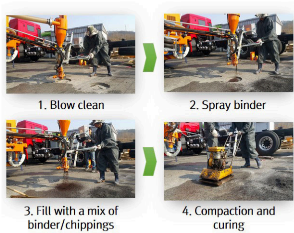
Fig. 10 Field Application of Spray Injection System
