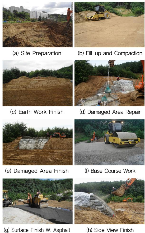
Fig. 22 Field Mock-up Construction
