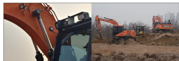
a) Installation of sensor modules b) Ground excavation
