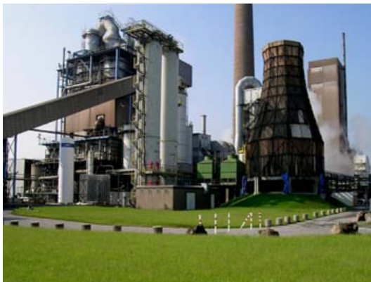
Fig. 2. Fluidized bed incinerator
