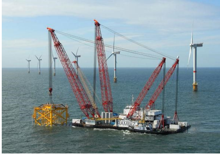
Fig. 1. Floating crane used for installing offshore structures
