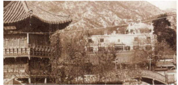
Figure 1. Gwanmungak(觀文閣) under construction, ref. the 20th commemoration exhibition of Korea-Russian treaty of army.
