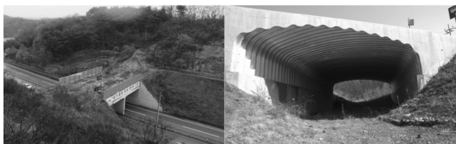
Fig. 1. Example of overpass (left) and underpass (right) wildlife crossing.
