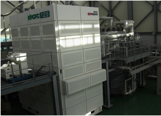
Fig. 6. 125 kW MCFC system
