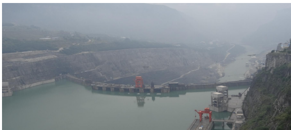
(a) Power station panorama
