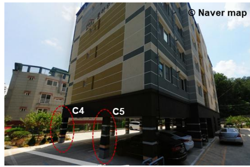
(a) The front view of F building
