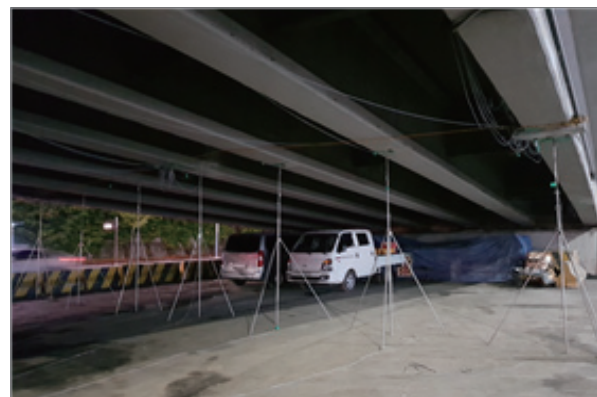
Figure 3. Overview of installed sensor
