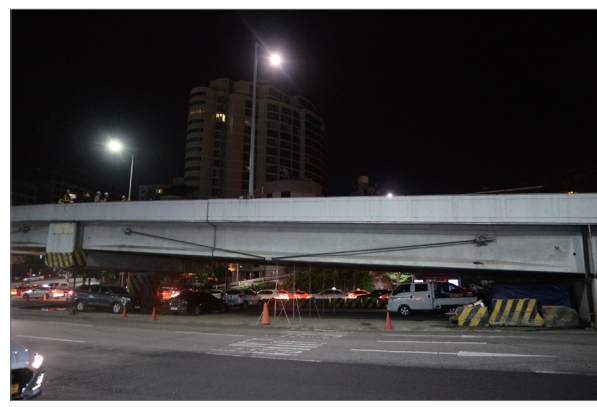
Figure 2. Overview of PSC girder bridge
