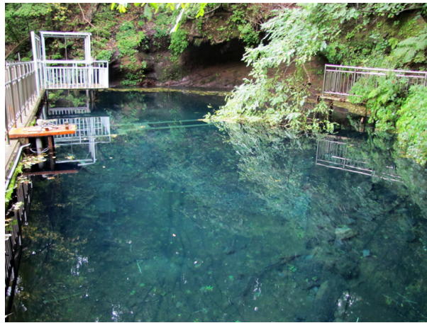
Fig. 3. The dam constructed at Yongchulso Spring.
