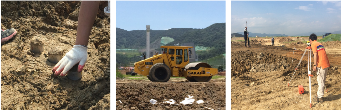
(a) Installation of containers measuring density of ground
