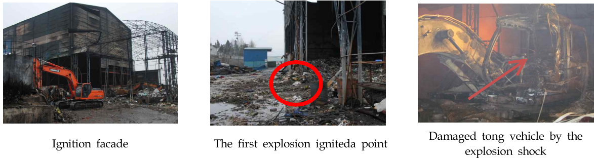
Fig. 3. Packaging waste explosives fire explosion accident scene
