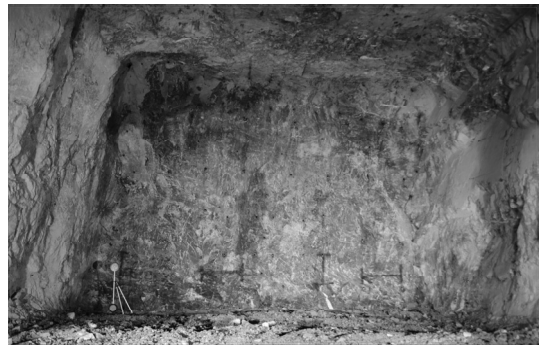
Fig. 1. Photograph of excavation face at Lv520.
