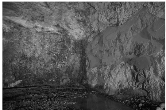
Fig. 10. Photograph of steeply dipping joints in test area.
