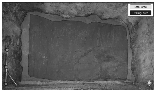
Fig. 6. Total area and drilling area at excavation face (fourth blast).
