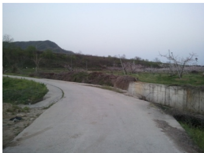
Fig. 1 Curve road where the rollover accident happened
