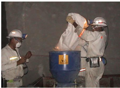
(a) Batching and mixing of TSL
