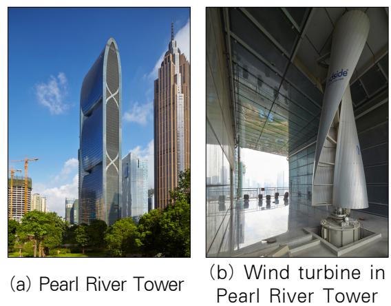
<Fig. 2> Pearl River Tower and wind turbine
