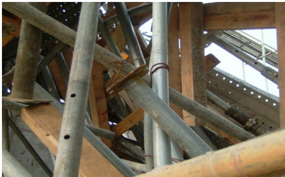
<Fig. 4> Misuse of vertical member connection
