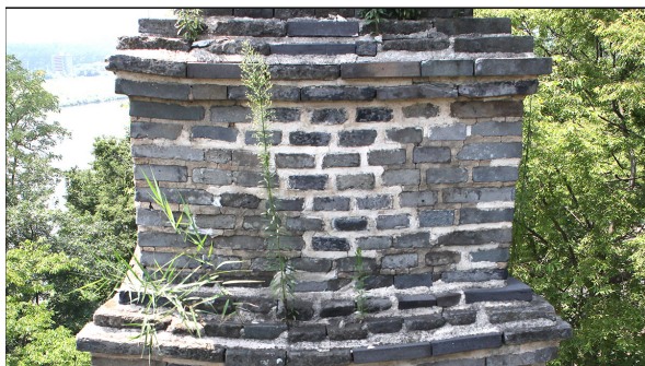
(Fig. 9) Joint of Silleuksa Pagoda
