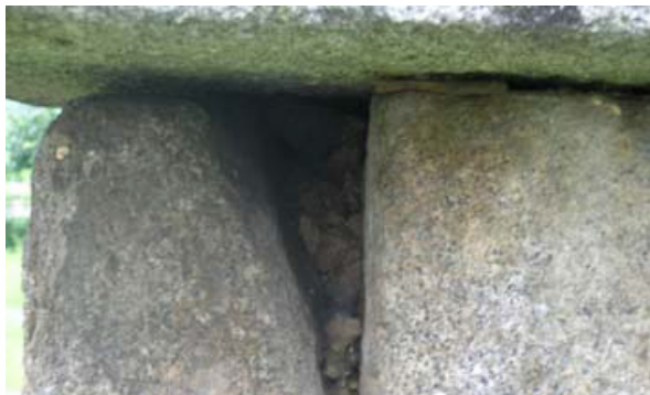
(Fig. 8) Infill material of Bongeopsa temple site pagoda
