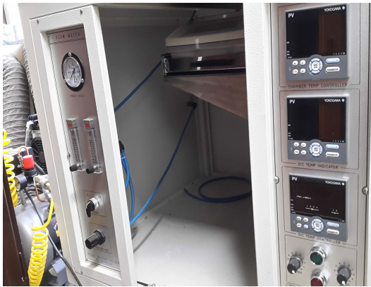
Fig. 2. Controller and weighing scales of the combustion furnace.
