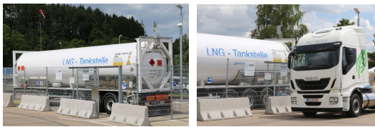
Fig. 6. Mobile LNG Fueling Station in Germany
