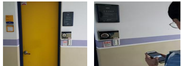
Fig. 12. Construction Field of Proposed System
