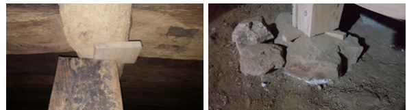
(b) Wood plates seated on the top and bottom of the altar
