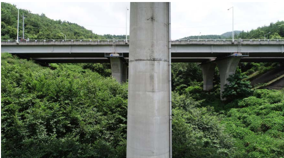
Fig. 1. Lateral view of the bridge pier
