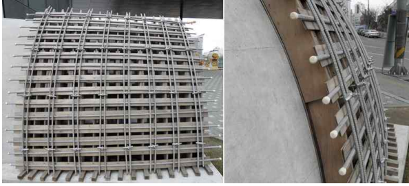
Figure 2. Timber forms(DDP, Lib Form)
