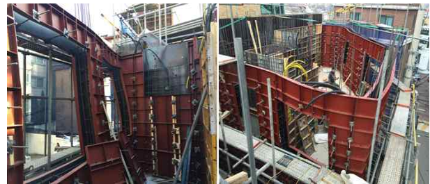
Figure 4. Steel forms
