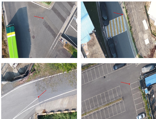
Fig. 12. Check Points of UAV
