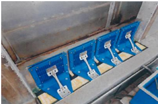
Fig. 7. After test specimen installation
