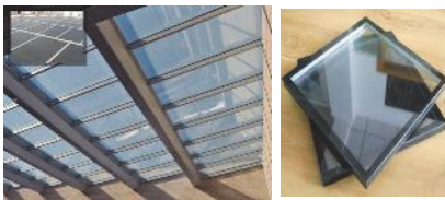
Fig. 8. Semi-transparent Double-glazed PV windows
