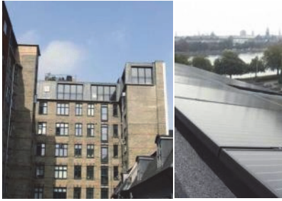
Fig. 7. Ryesgade 30 A-C(Copenhagen 5 story 32 apartment house from 1896), Facade and solar cell roof (Smart Architectural Retrofitting)
