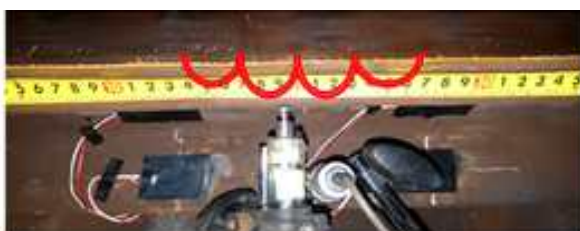
(c) Photos of corrugation on tested section
