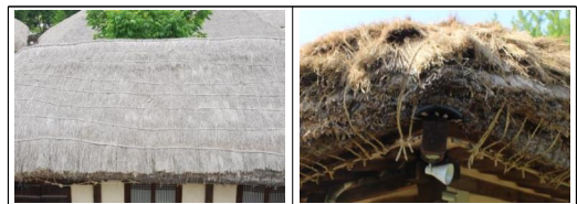
Fig. 12. Present Conditional of Straw-rope and Angle Rafter Maguri
