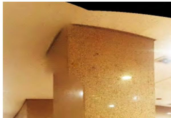
Column in the building
